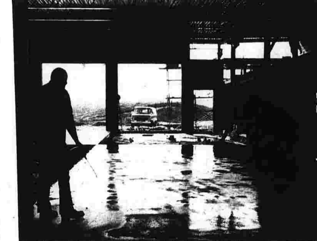
Firehouse progress in South Windsor Work is moving right along on the new South Windsor firehouse on Ellington Road. A construction worker is shown pouring one of the huge expanses of cement. (Herald photo by Pinto)
